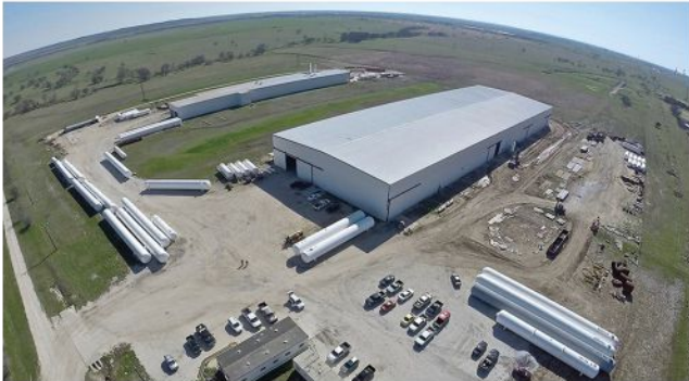
McGregor, TX 170,000 square foot fabrication facility
